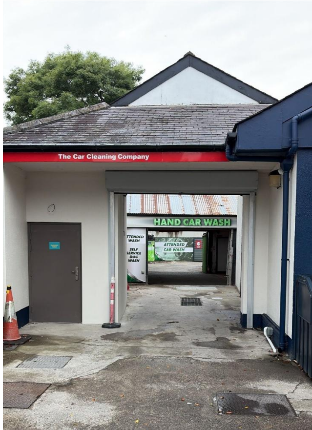
Fig No.10 Access from the service station to the car wash – as viewed from the service station.
