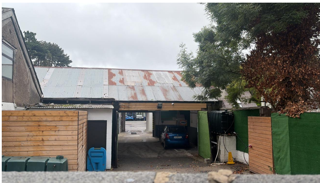
Fig No.9 View from Westminster Lane into the site over the boundary wall showing the link to the site via the structure at the east side of the site.
