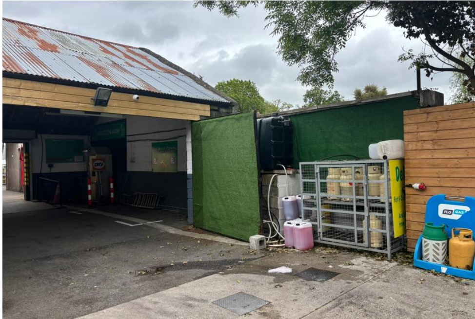
Fig No.5 Photograph of the access from the service station.
